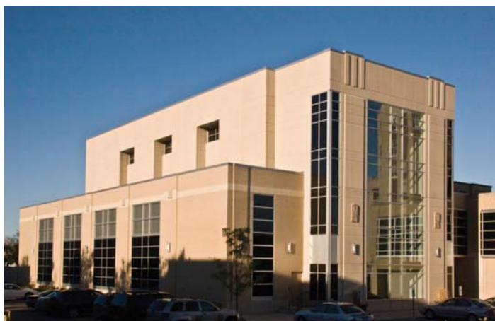
Rockford Register Star Press Addition - Rockford, Illinois
