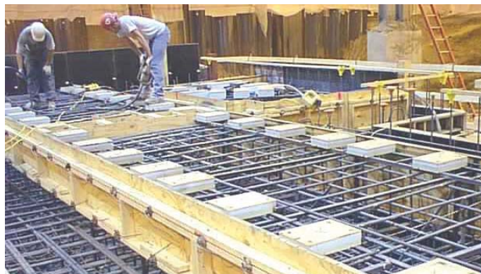
Caterpillar C175 Machine Foundation
